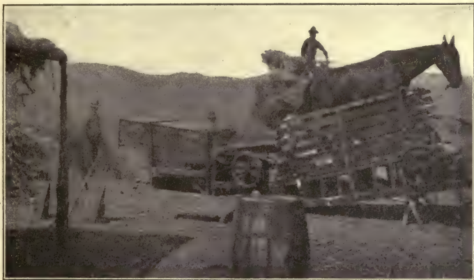
FIG. 100. Using treadmill for threshing grain from small plants on one of the Utah experimental dry-farms.
