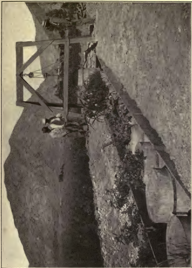
FIG. 5. Weighing pots to determine the amount of water required for the production of plants. Utah, 1901.
